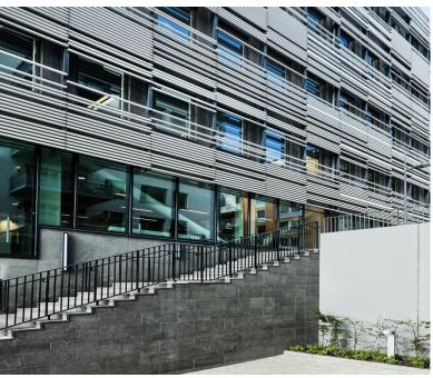
The sun-screen system is synchronised with Skanska's cooling system
