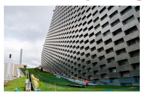
440,000 tons of waste is yearly converted by furnaces, steam and turbines into clean electricity and heating for 150,000 nearby homes
