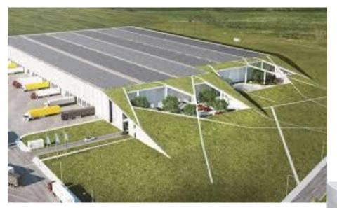
Offices located under a green roof will not heat up in summer, and will save heat energy in winter, reduce the load on the rainwater drainage system
